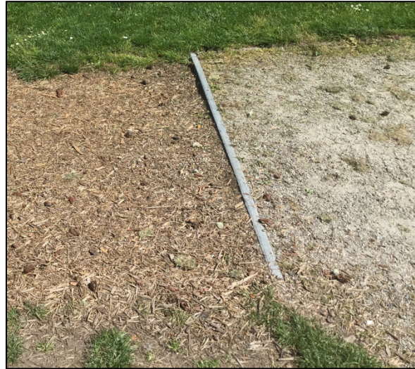
Figure 9 Path transition tripping hazard
