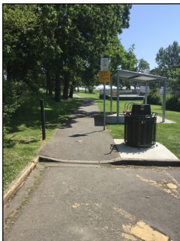
Figure 10 Excessive lip to curb cut
