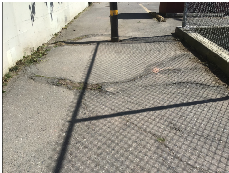
Figure 8 Cracked and lifting asphalt
