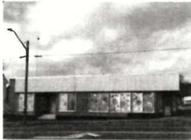
view of building at Hillside Ave. (south side)
