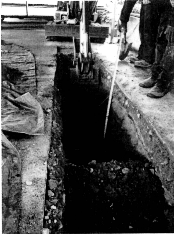
Picture #6: Two 3cm Cedrus roots were pruned 1m north of the hydro pole. An additional eight 1cm diameter roots were encountered north of the hydro pole.
