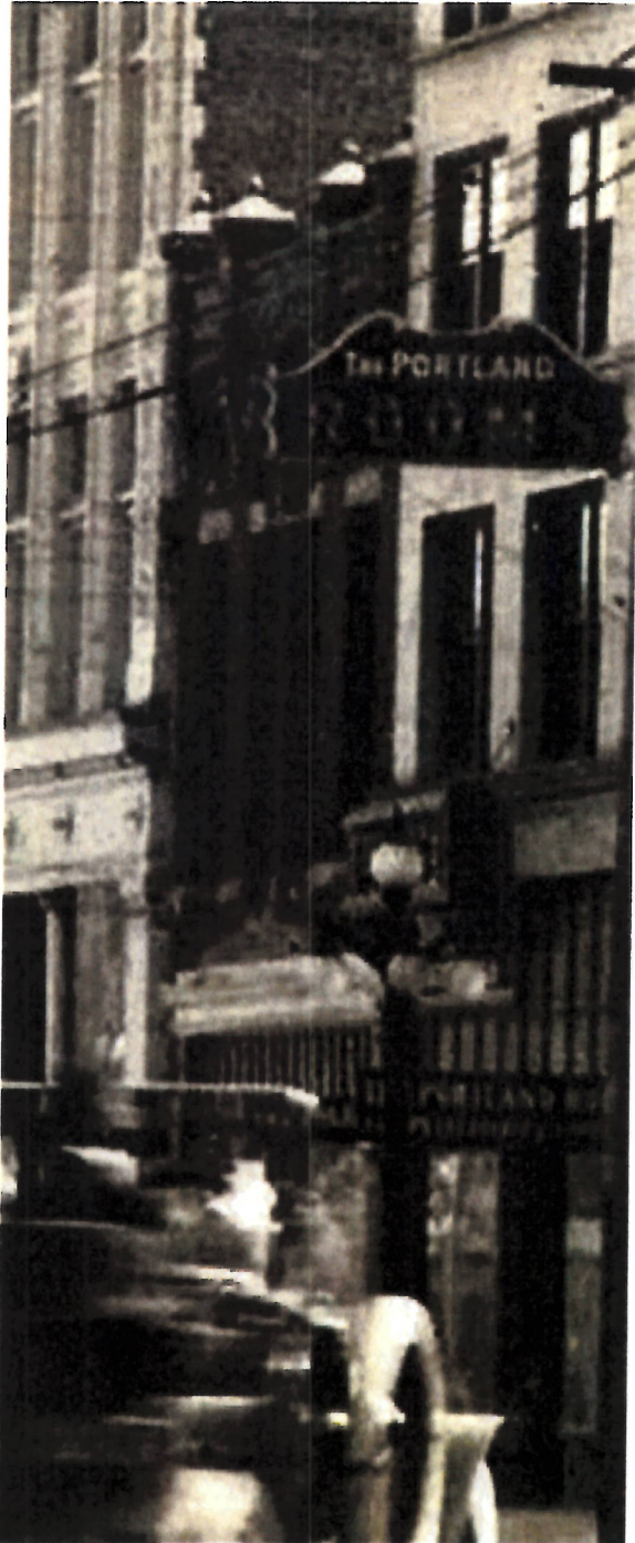
Detail photo showing historic front facade of the Hall Block and adjacent buildings along Yates Street. Note original storefront with transom ribbon, architectural metal cornice, and window openings with sandstone sill. (BC Archives, E-02737)
