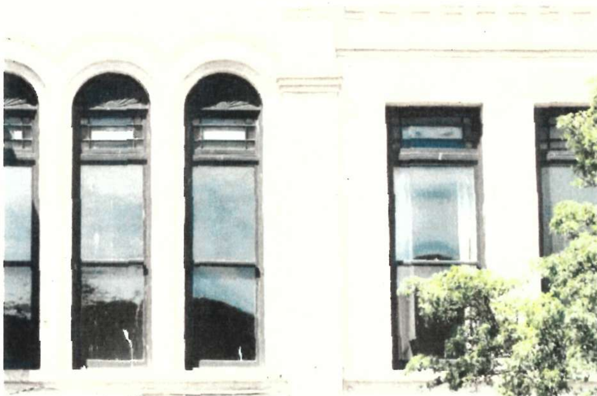
Detail photo partially showing existing window openings, with surviving original wood window assemblies at the upper level of the historic street facade.
