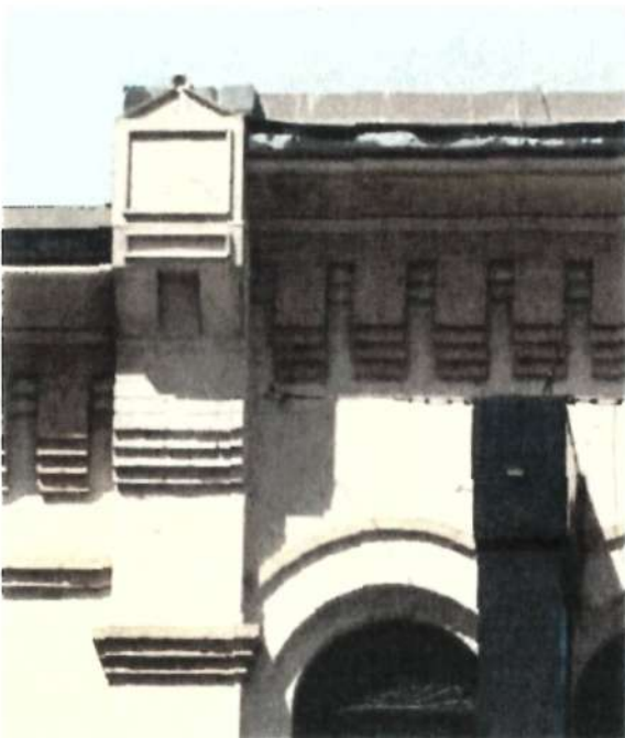
Detail photo showing typical condition of architectural brickwork detailing and metalwork along parapet level.
