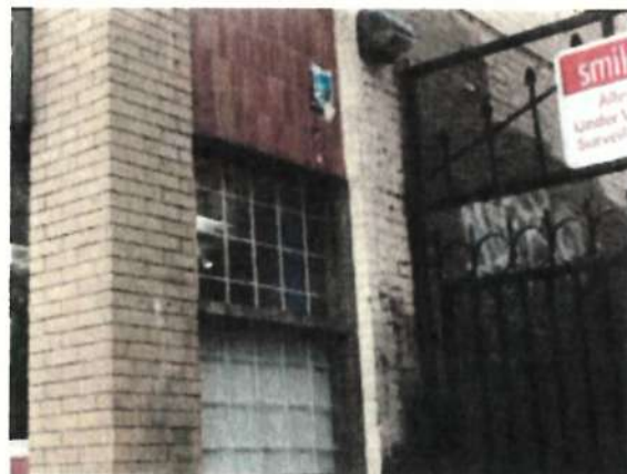
Photo showing storefront return, and partial masonry wall along the laneway elevation to the east; note tilework at the storefront transom that are not original and should be removed.
