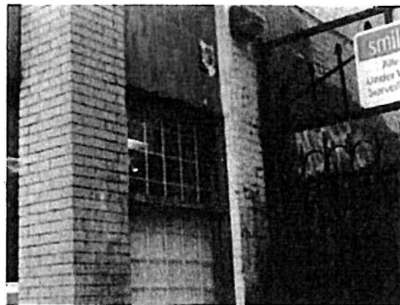
Photo showing storefront return, and partial masonry wall along the laneway elevation to the east; note tilework at the storefront transom that are not original and should be removed.
