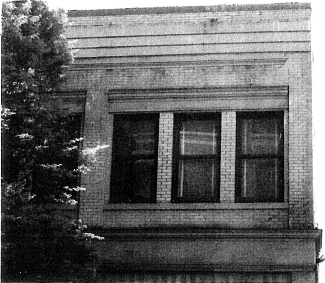
Photo showing partial exterior masonry wall above the storefront. Note typical deterioration of masonry wall.
