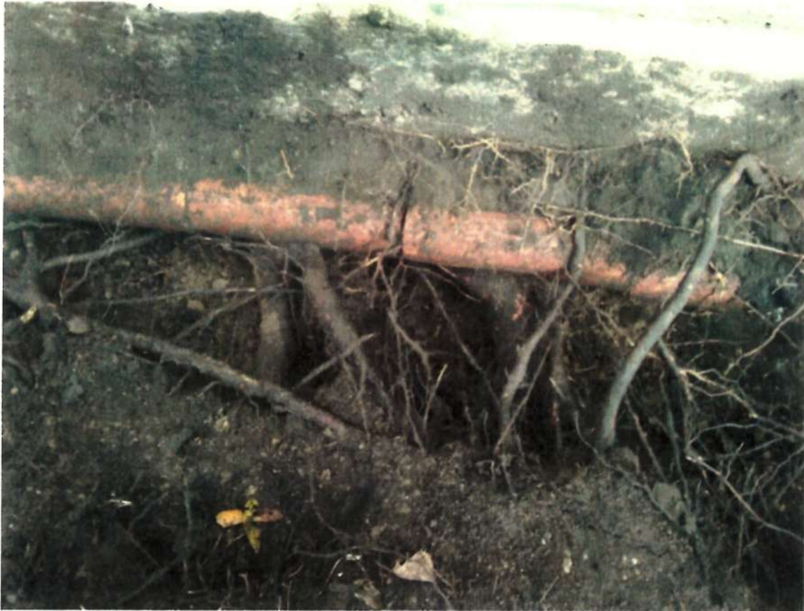
Photo 5. Showing exposed roots from maple hitting perimeter drain and foundation
