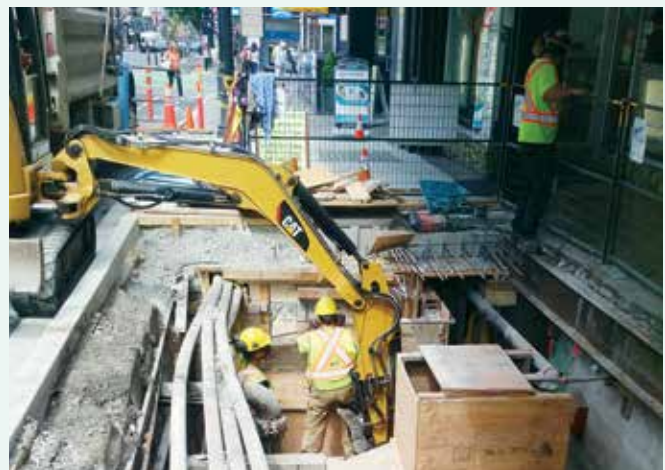
City carpenters working on Fort Street.
