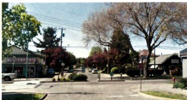
Above: Directional diverter - Kings/Shelbourne
