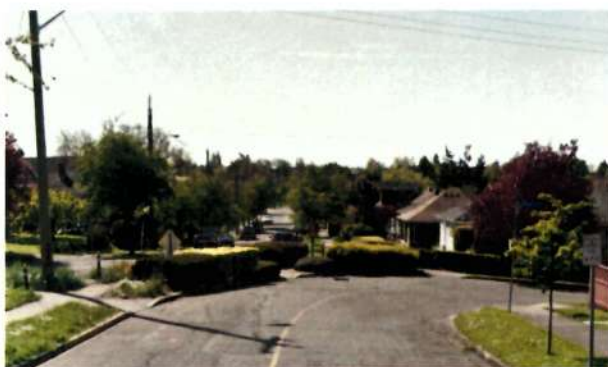
Above: Permanent diagonal diverter – Blackwood/Kings
