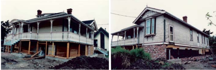
Structure raised and new foundation with finished basement in 1990
