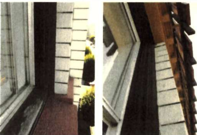
Details of the wooden frames and mouldings on the main facade.
