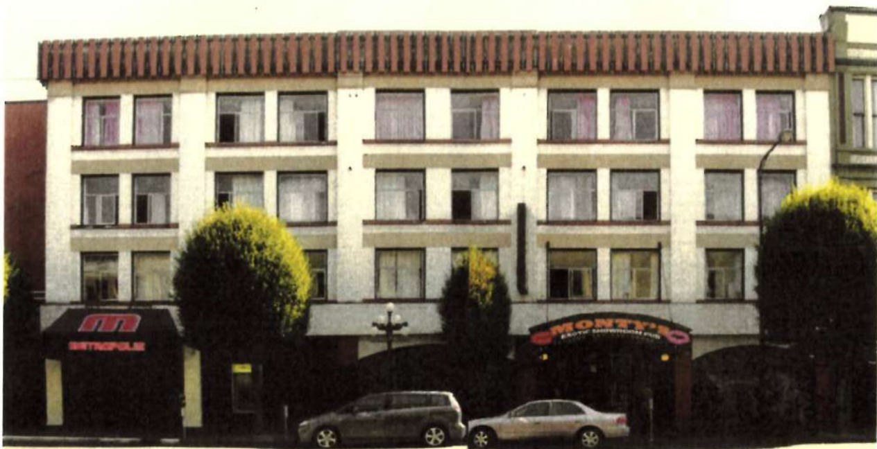
Historic facade viewed from Government Street
