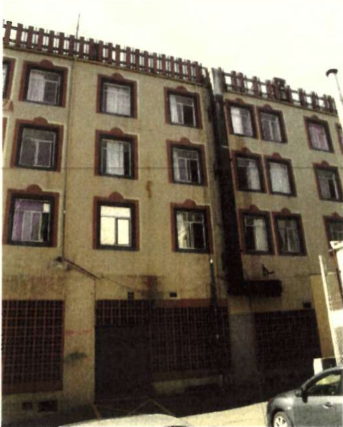
East elevation with stucco finish and breeze blocks.
