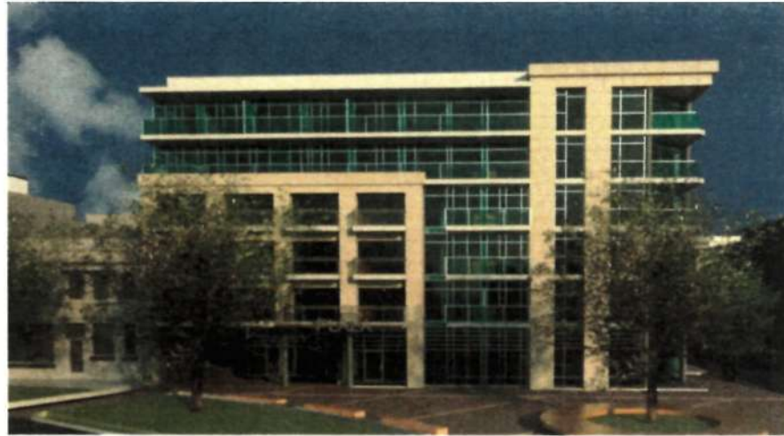
6 West View to South
