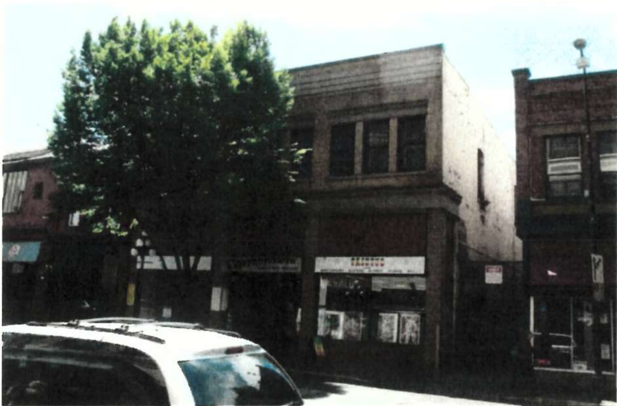
Top (right) and bottom: Photos showing partial front and side (laneway) elevations, as viewed from Johnson Street.
