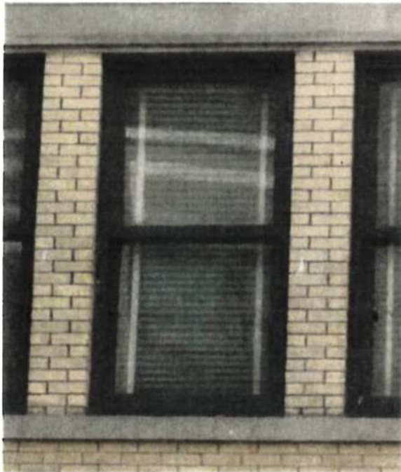
Typical existing condition of double-hung wood sash window at upper level.
