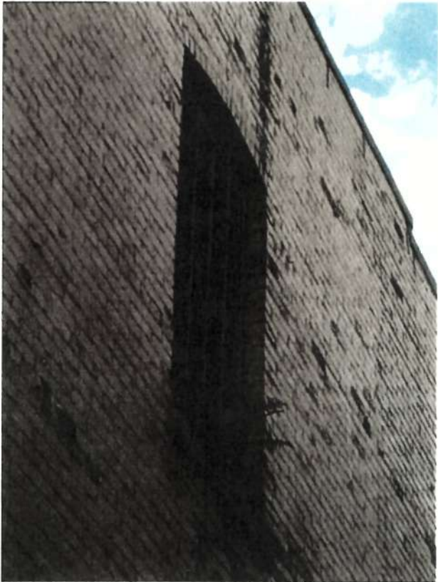
Upper West Wall Semi-Arched Windows
