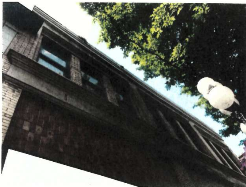
Upper North Facade
