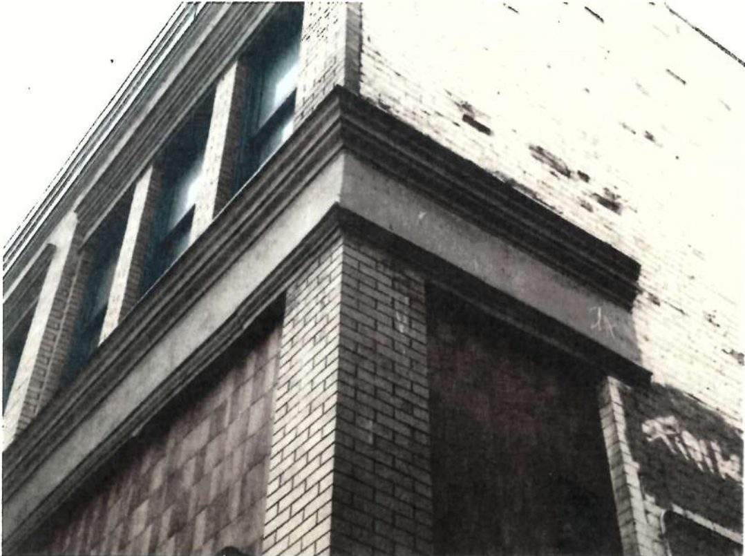
Upper Cornice Return
