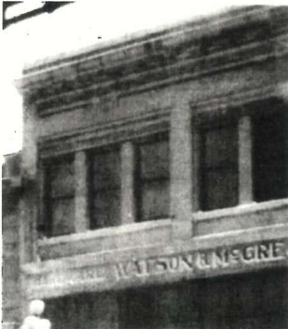
Detail photo showing project metal cornice at parapet level, and the storefront cornice with signband at the lower street facade, circa 1913 [Collection Nancy Davis; Hallmark Society Files]
