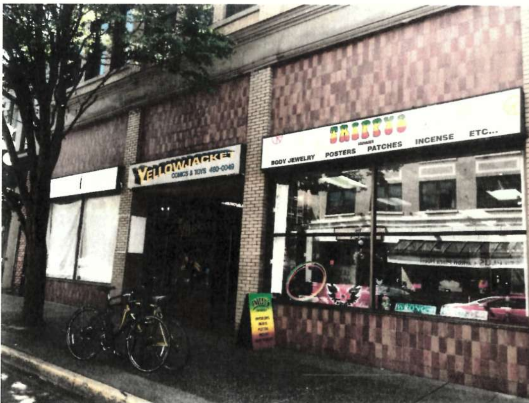
Lower North Façade with Central Entry
