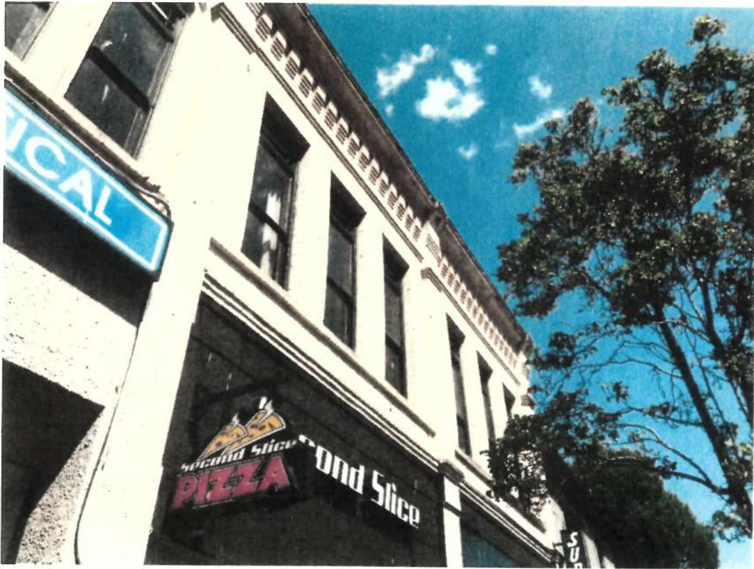
Upper Right Bays with Double Hung Windows and Corbelled Brick
