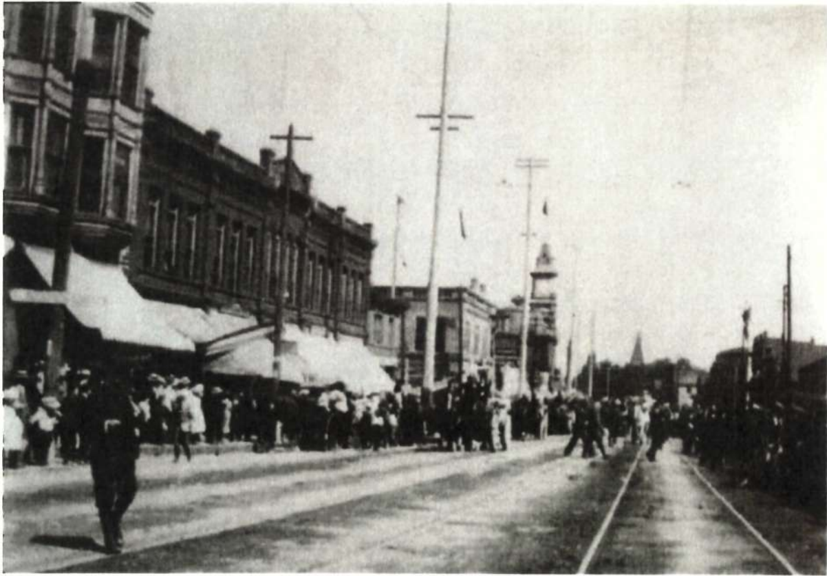
View From Douglas Street Looking West - Morgan Block - 1890s [City of Victoria Archives M09112]
