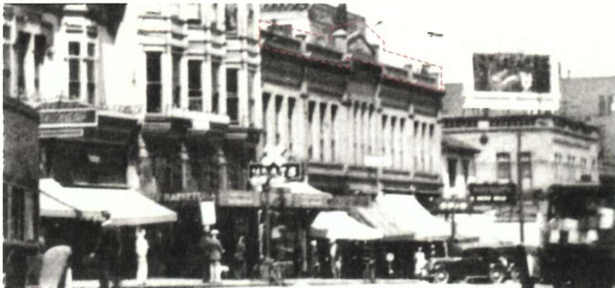
Detail photos showing original parapet wall (outlined in red) that is no longer extant.
