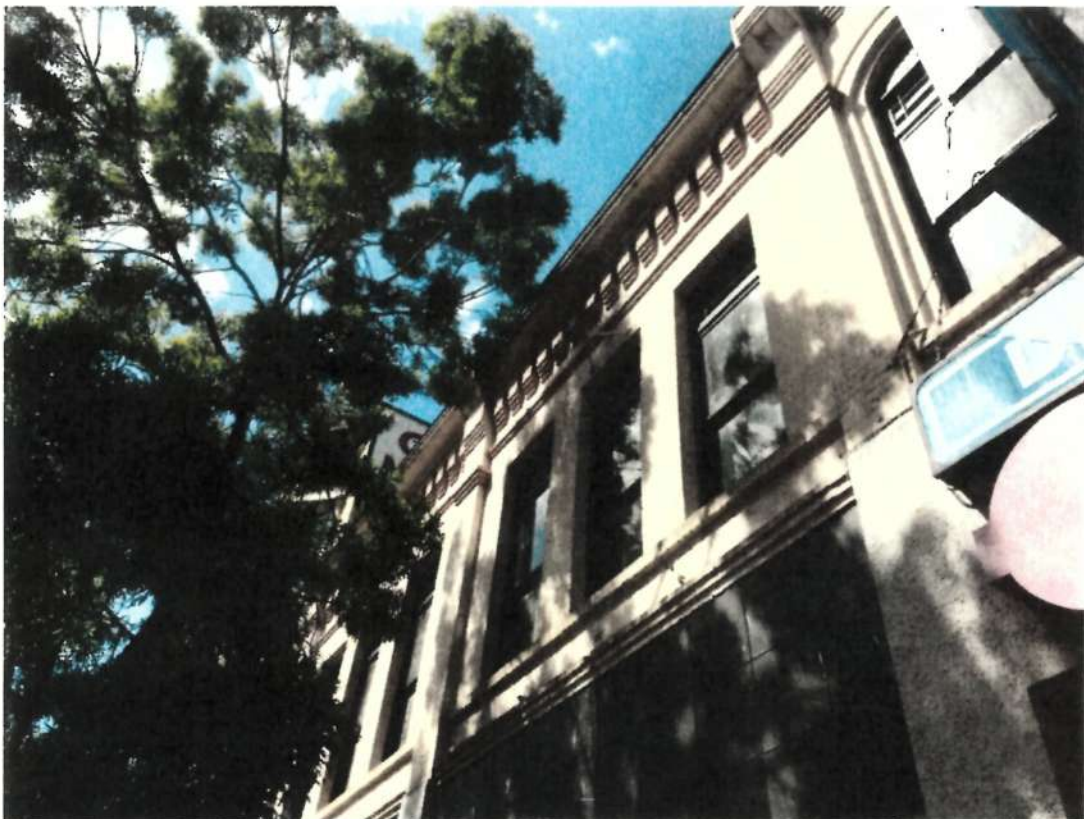
Upper Left Bays with Double Hung Windows and Corbelled Brick
