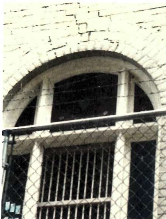
Detail photo showing tripartite wood window assembly. Note semi-circular arched transom with surviving original multi-pane leaded wood sashes in true divided lights.
