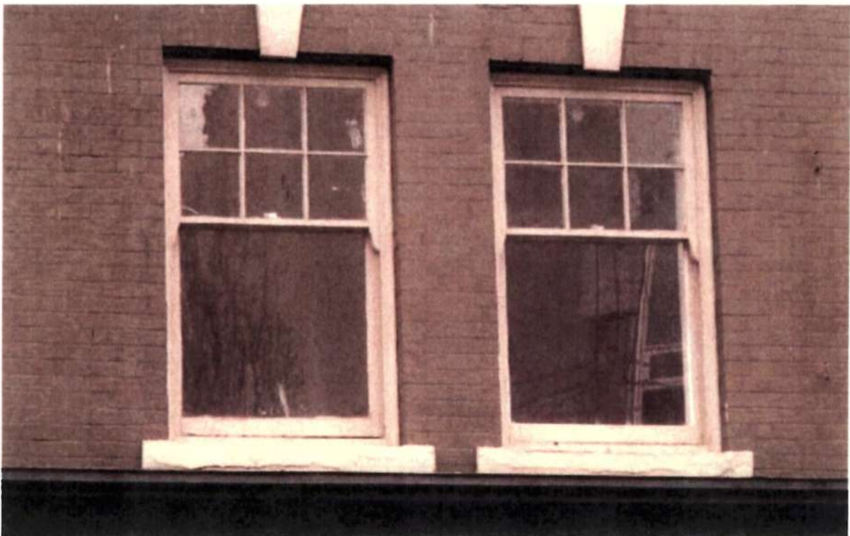
Two of the four surviving original double-hung wood sash windows at the upper level of the historic front facade. Note multi-pane upper sashes in true divided lights, with true integral sash horns.
