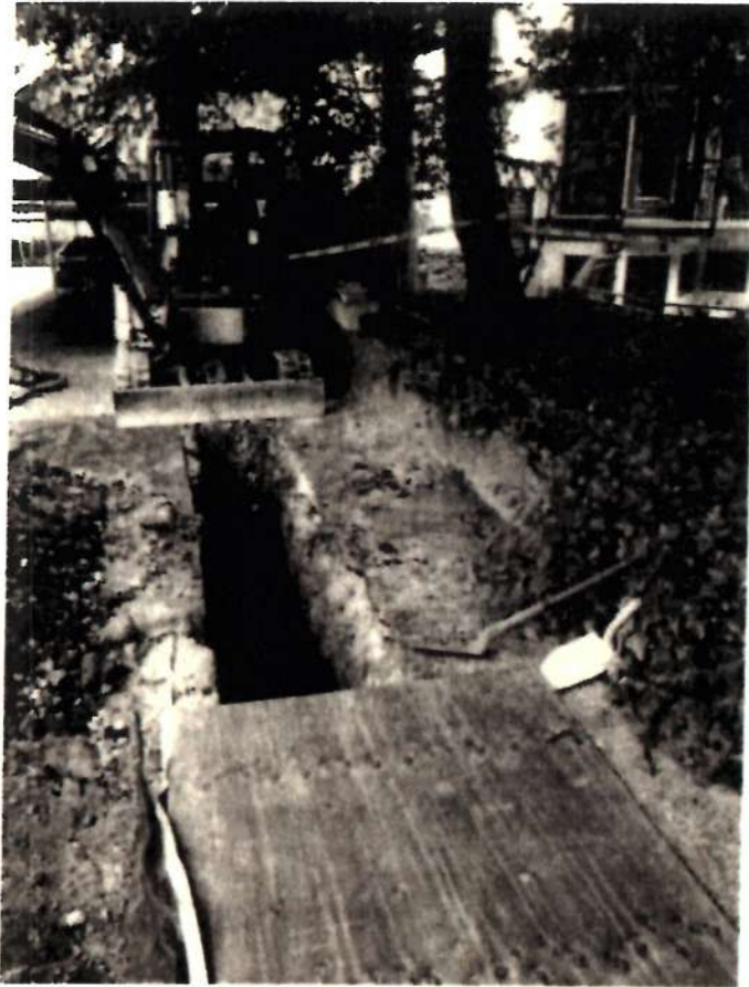
Picture #3: A 60cm wide trench, 90cm in depth, was excavated 60cm west of the retaining wall.
