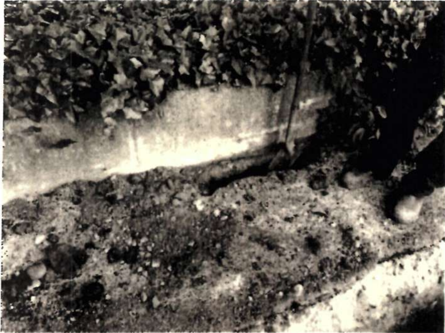
Picture #2: A small area of uplifting pavement was removed west of Deodar Cedar NT9. A 5-6cm diameter root was encountered directly underneath the pavement.
