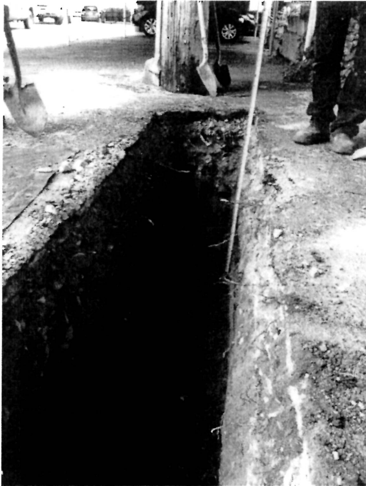
Picture #4: Several small roots, 1cm or less in diameter, were encountered up to the hydro pole.
