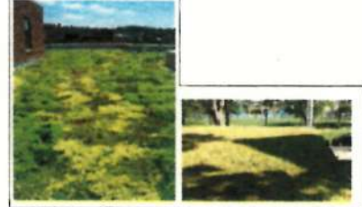
4. Sedum green roof above parking and bike storage.
