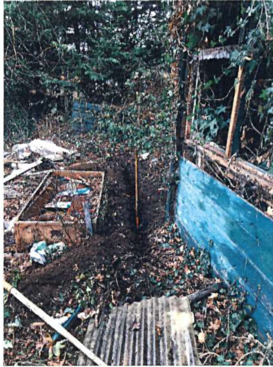
We hand-dug a 2.5m long trench 1.5m from the base of the 83cm DBH Garry Oak (#450), where we anticipate excavation will occur to for construction of the building on lot 2.
