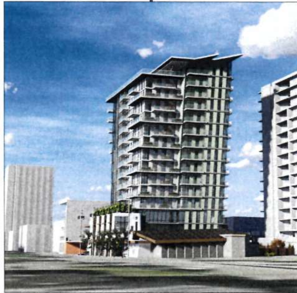
STREET VIEW, SOUTH EAST
