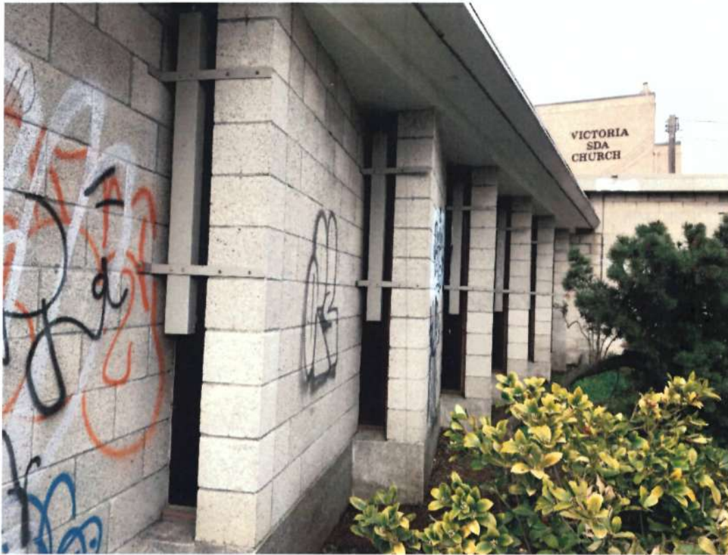
Saw-tooth splayed concrete walls
