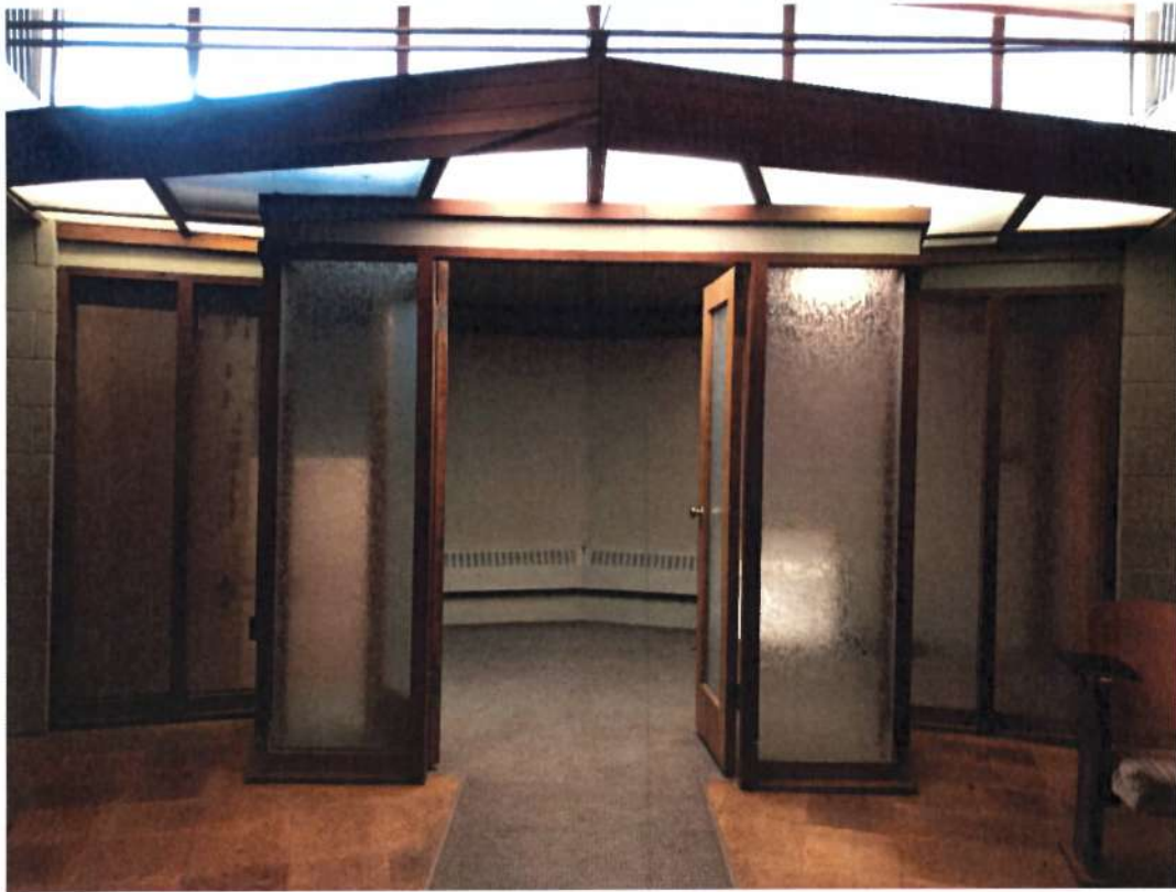
Inner vestibule and projecting canopy
