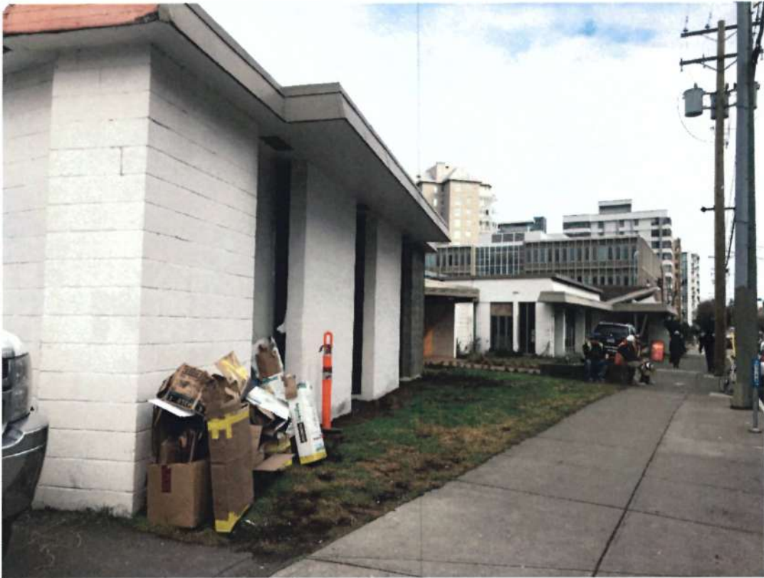
View on Johnson Street looking east from west corner of the 1961 addition
