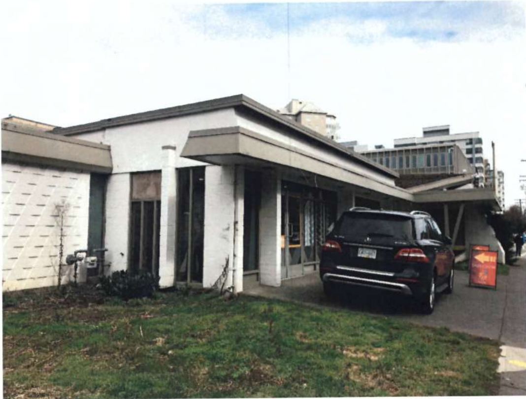
1961 Addition (View of Chapel wall buttress in the distance)
