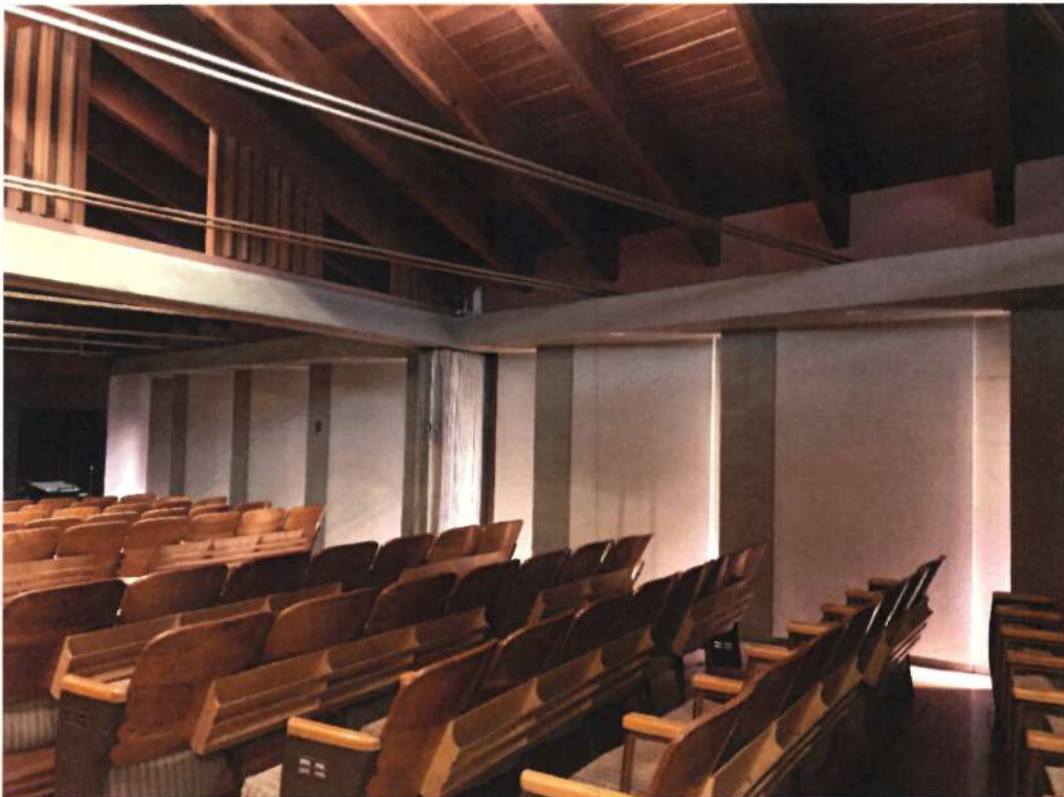
Interior east wall
