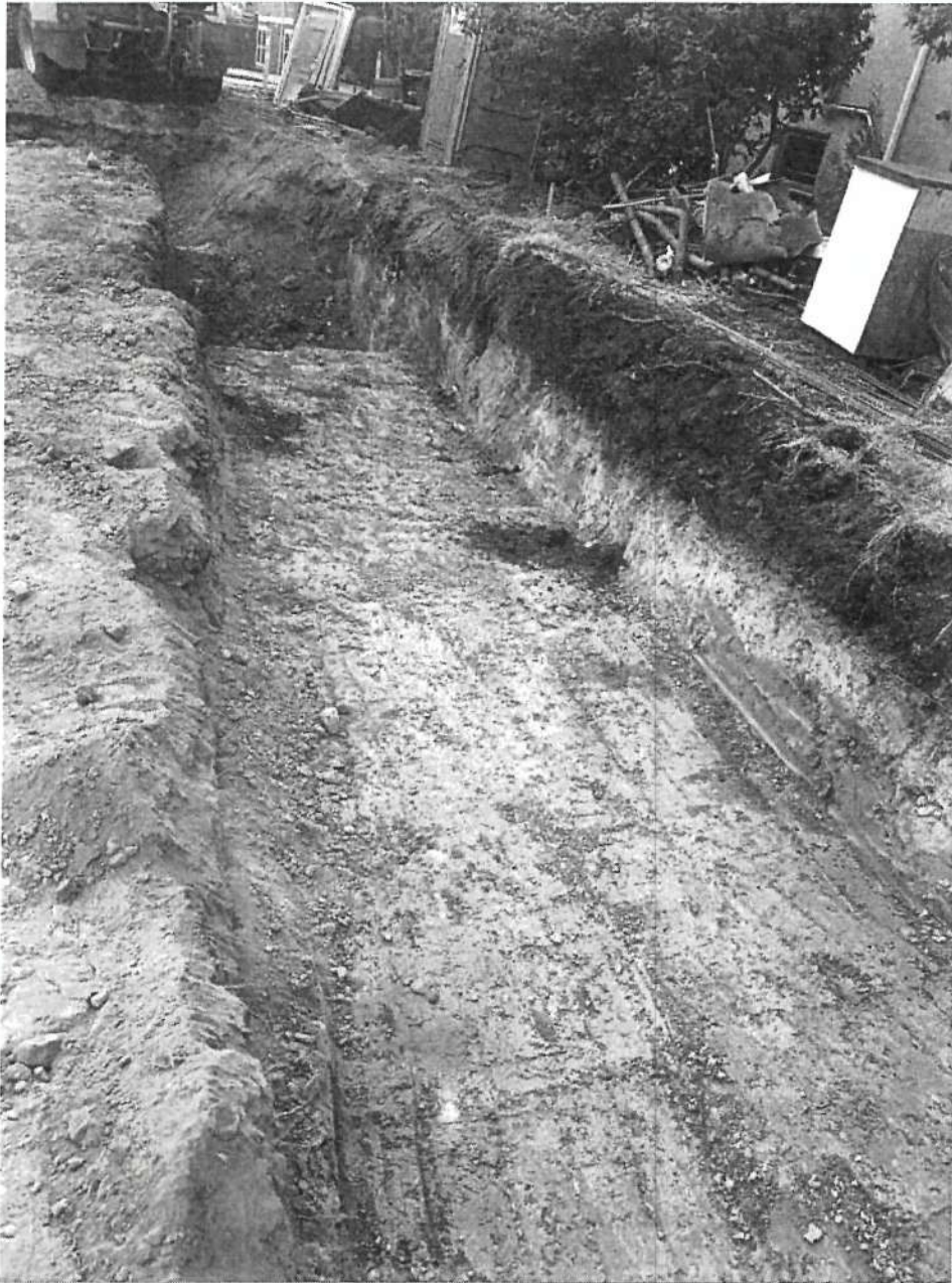
Picture 2: View of excavation from second angle showing no large roots exposed (picture supplied by client).
