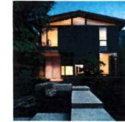
Clear finished wood accents at entries and soffits in conjunction with native painting and dark batten trim. D'Amey Jones Architect, Vancouver, BC
