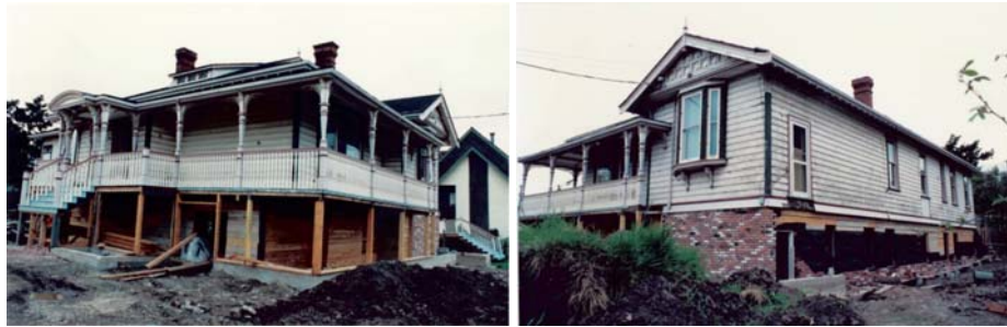
Structure raised and new foundation with finished basement in 1990
