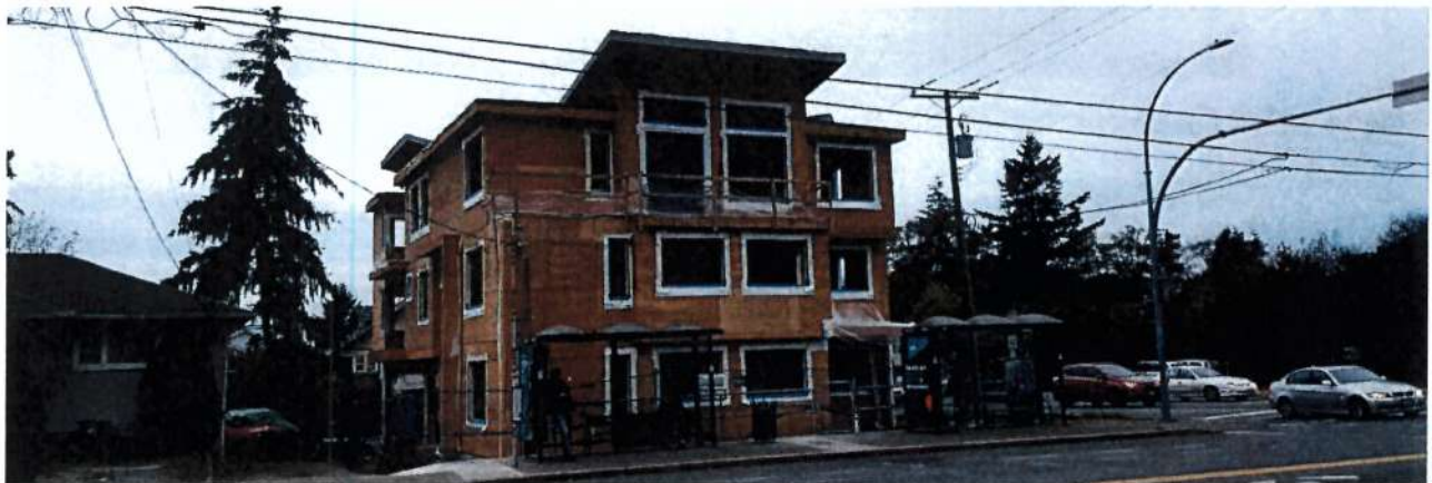
Fig 23. Three storey apartments being constructed on Bay St and Richmond Ave
