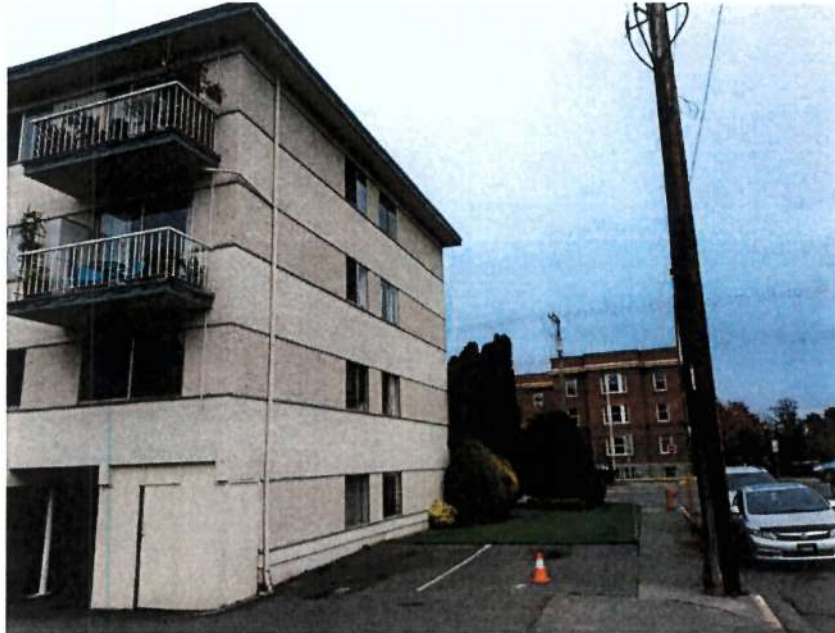
Fig 16. Apartment complex (foreground) Jubilee Hospital Heritage Building (Background)
