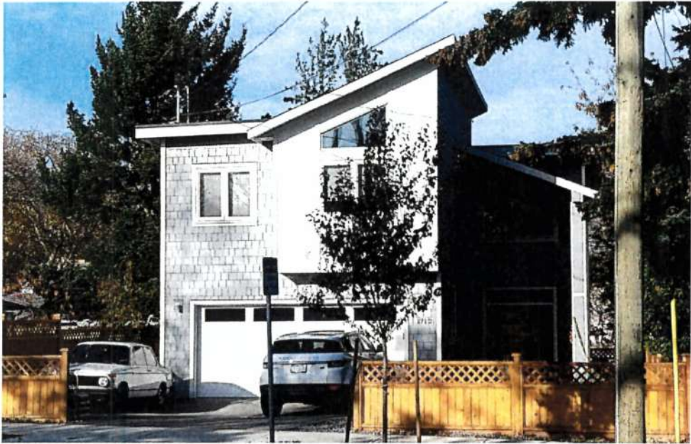
Fig 24. Newly constructed low slope roof home on Haultain Street
