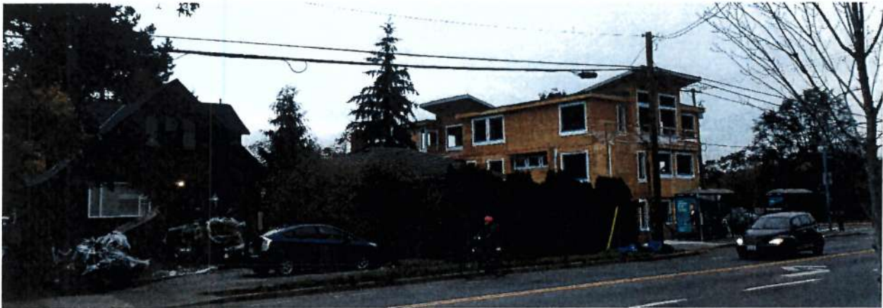
Fig 22. Three storey apartments being constructed on Bay St and Richmond Ave
