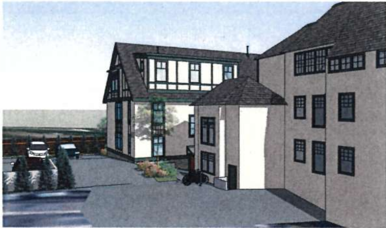
View from Parking Lot looking East
