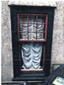
Existing Window Photos
