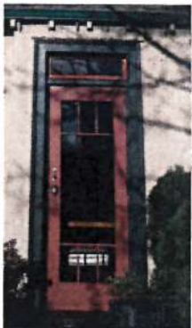
Abigail's Existing Door Photo
