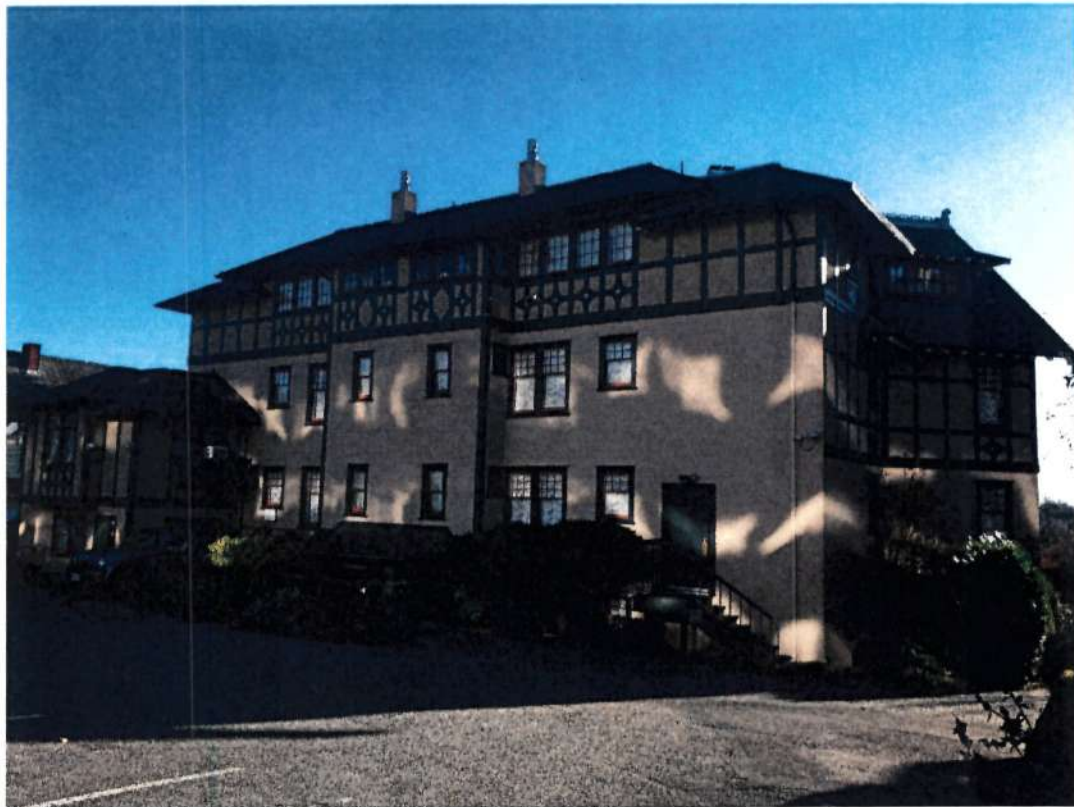
North Rear Façade
