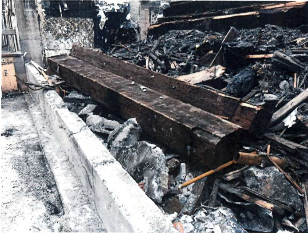
Remnants of heavy timber structural members
