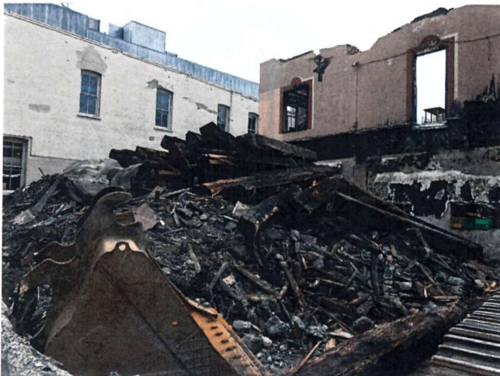
Remnants of heavy timber structural members
