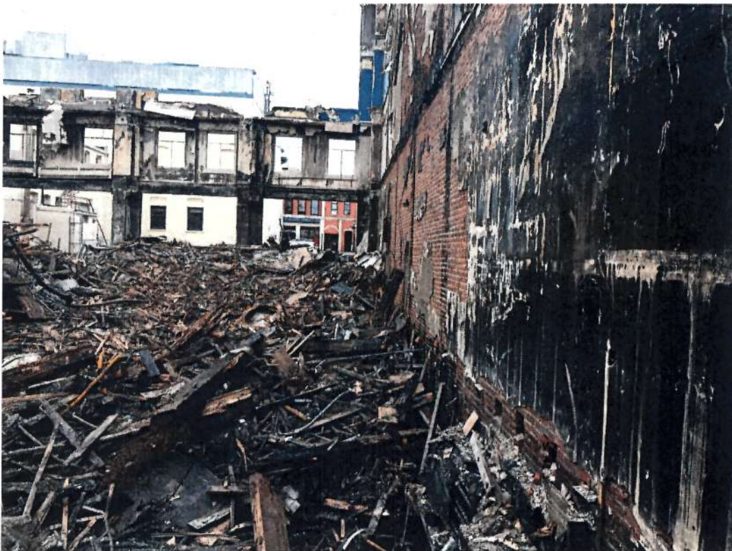
Looking east along north wall of 1411 Government Street
