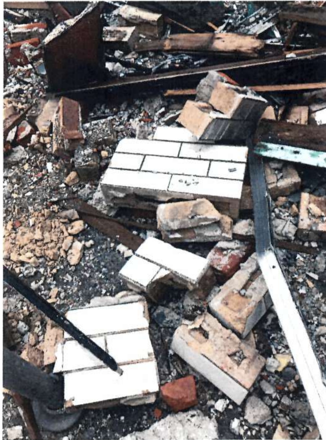
Remnants of white glazed brick from front façade
