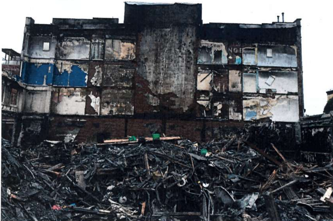
North wall of adjacent 1411 Government Street
