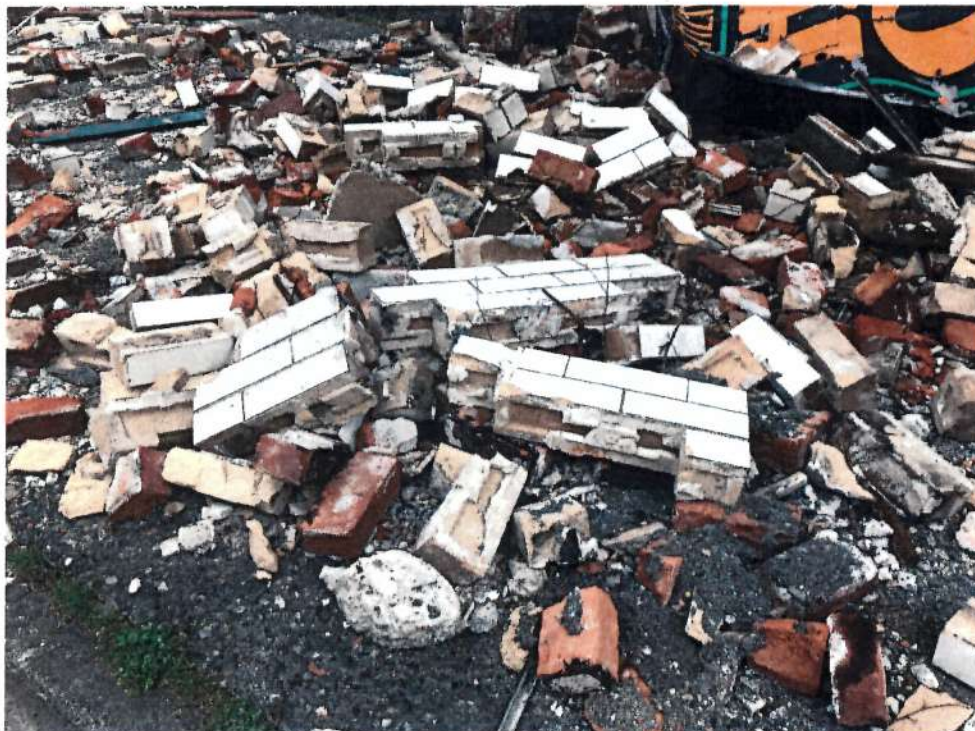
Remnants of white glazed brick units from front façade
