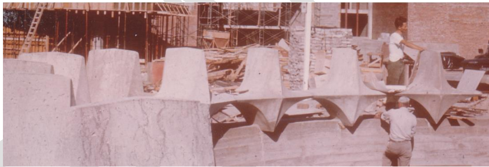
Centennial Square Fountain under Construction
