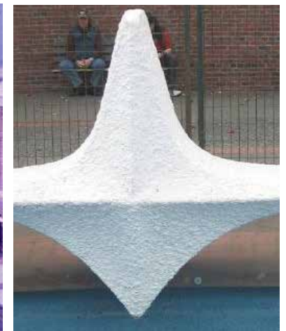
Tiara covers in Stucco
