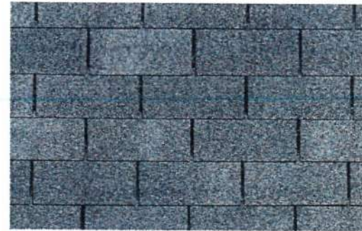
GRAY ASPHALT SHINGLE ROOF
