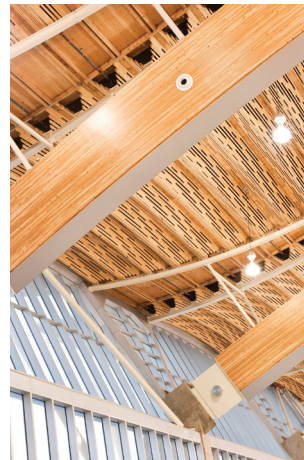
The 330 foot long Glulam Mass Timber beams at the Richmond Speed Skating Oval in 2009.
