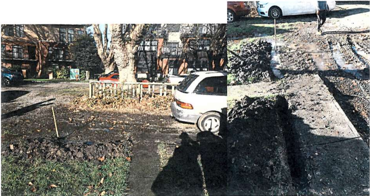
Photos 4 and 5: Excavation adjacent to London Plane #3. Compaction as a result of vehicles is already present on-site.
