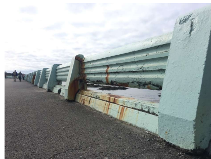
FAILURE OF STEEL REINFORCEMENT: JULY 2019
