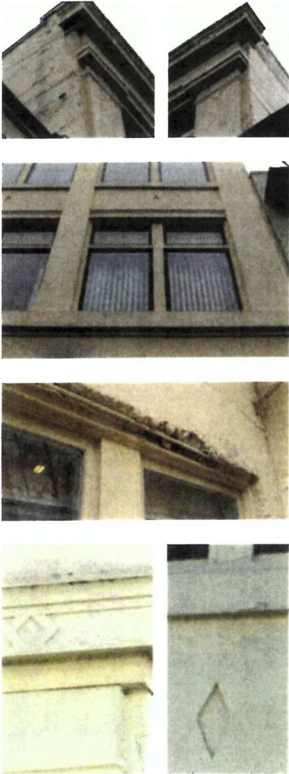
Photos showing typical deterioration of the exterior walls.
