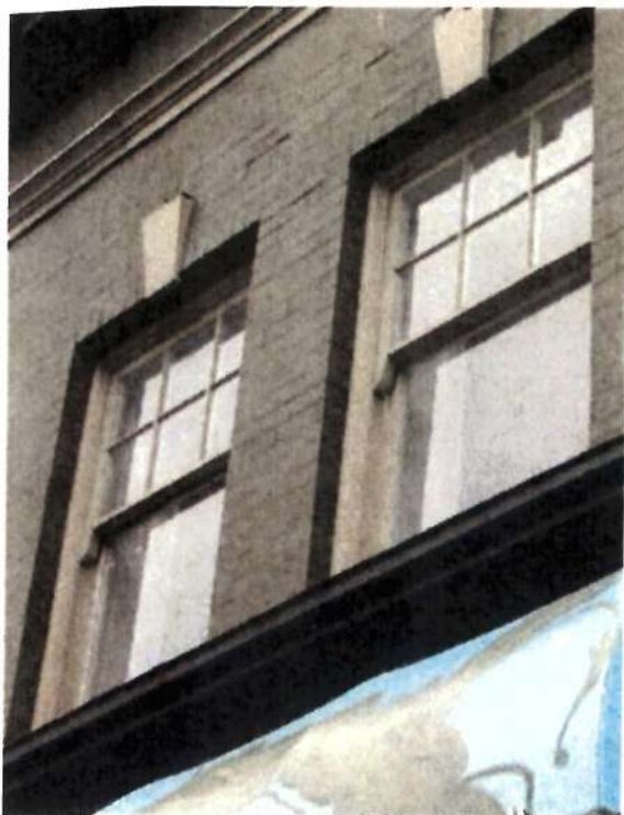
Detail photo of original double-hung wood sash windows at the upper level of the historic front facade.
