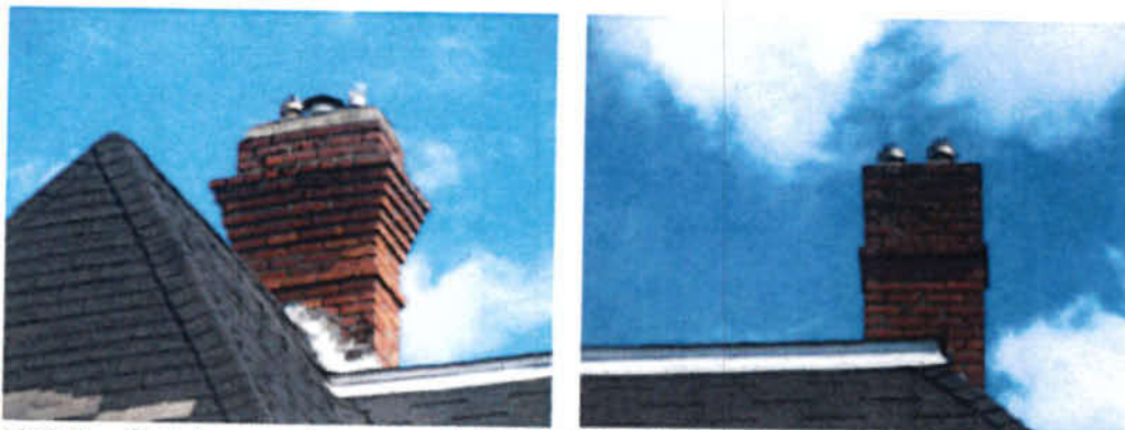
1139 Burdett Avenue chimneys: Original design left; to be rebuilt, right. Both chimneys will be taken down to roof and rebuilt to original design.
