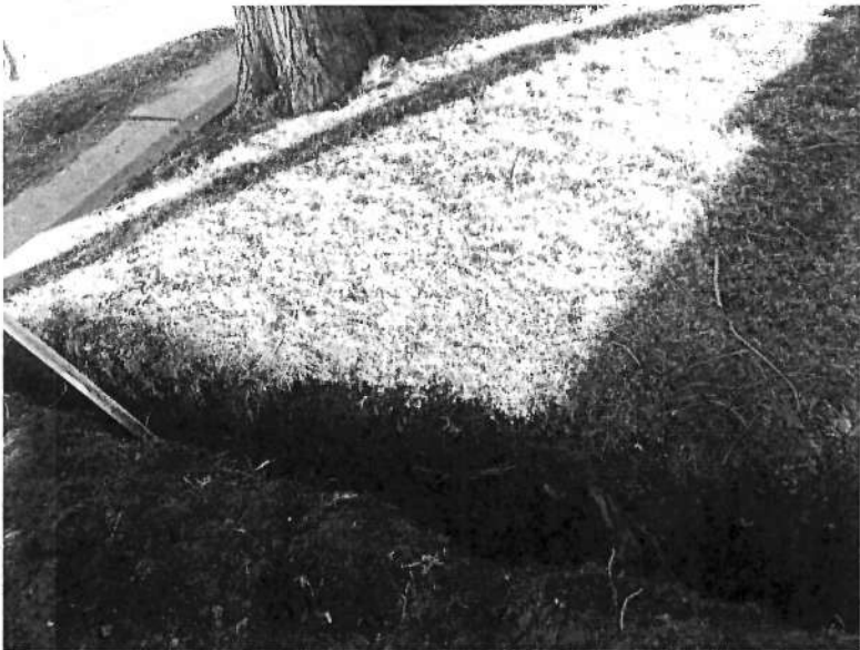
Photo 4: 2.5cm retained root on the right side within the trench.
