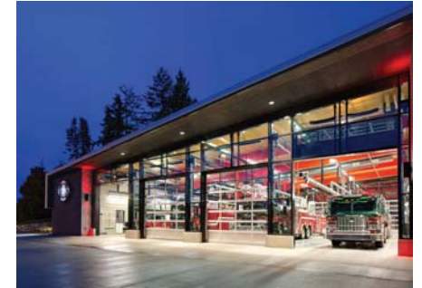
CONTEMPORARY FIREHALL VIEW ROYAL PUBLIC SAFETY BUILDING HCMA ARCHITECTURE AND DESIGN VIEW ROYAL, BC
