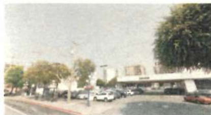
PHOTO - EXISTING VIEW NORTH FROM YATES
