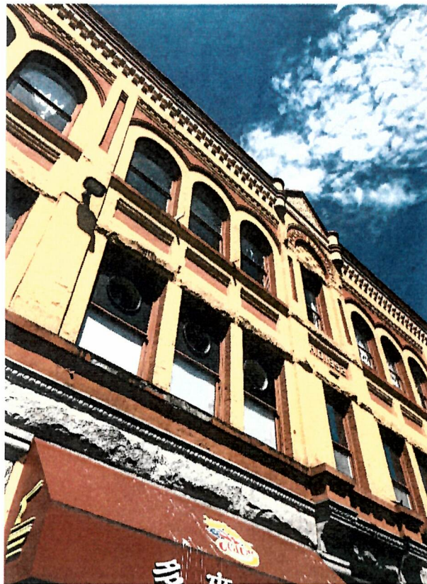
Arched Windows on Upper Storey
