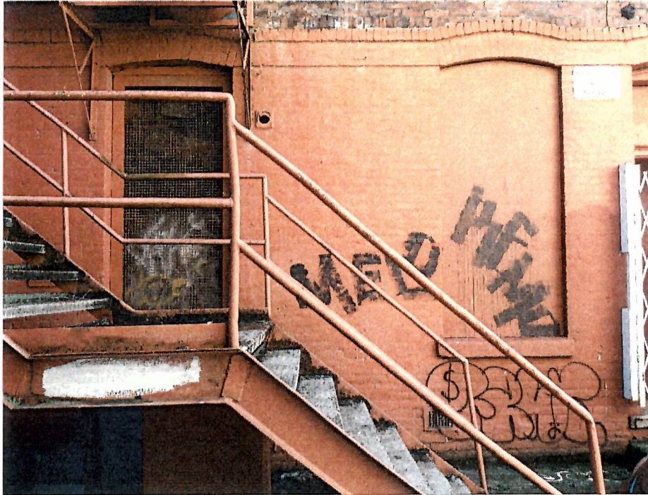
Rear elevation close-up
