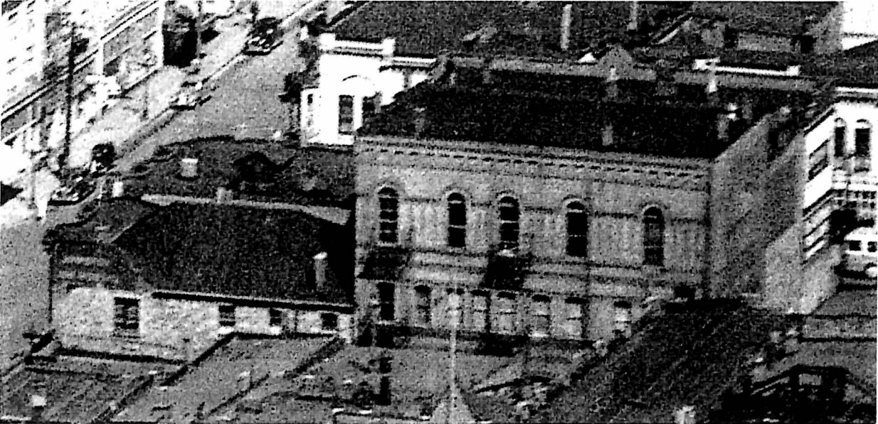
Victoria 1947 BO-47-1455 detail showing alley elevation. Note that the hipped roof of the Carriage Factory is still visible. It was later raised and flattened to match the roofline of the First Duck's Carriage Factory, and the stone wall extended upward in brick.
