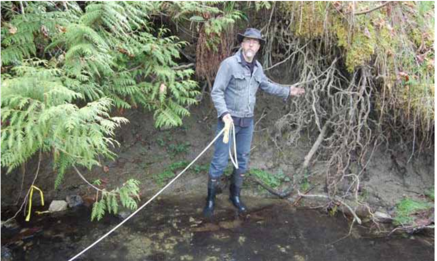
Photo: Stormwater erosion at Douglas Creek. Friends of Mount Douglas Park Society website: http://www.mountdouglaspark.ca/PhotoAlbums/Douglas%20Creek%20Storm%20Surge%20Erosion/index.html?delay=2&fullscreen=yes
