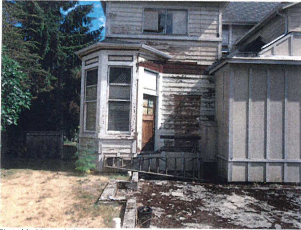
Five-sided bay window at SW corner of the house (rear view). This bay window contains original upper stained glass panels in each window. [Aluminum-framed window above will be replaced with wood sash]
