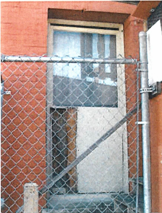
Below: Window on ground floor of rear façade with missing glass and loose upper sash.
