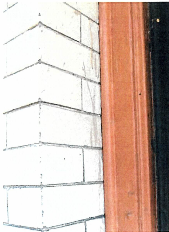
Above: Typical brick damage of chips and paint on brick face from painting adjacent wood elements, present on both "street" façades.
