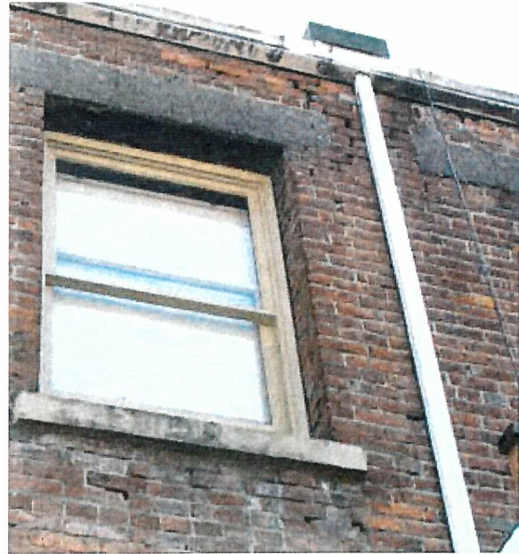
Above: Mortar loss, distortion of brick, and staining on rear of building likely caused by overflowing gutters and undersized downspout.
