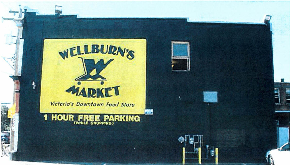
Above: Painted brick of the north façade. Paint is a later intervention and limits assessment of underlying brick. Surface damage to some brick and mortar loss present in areas at base of wall at approximate height of car mufflers and bumpers.
