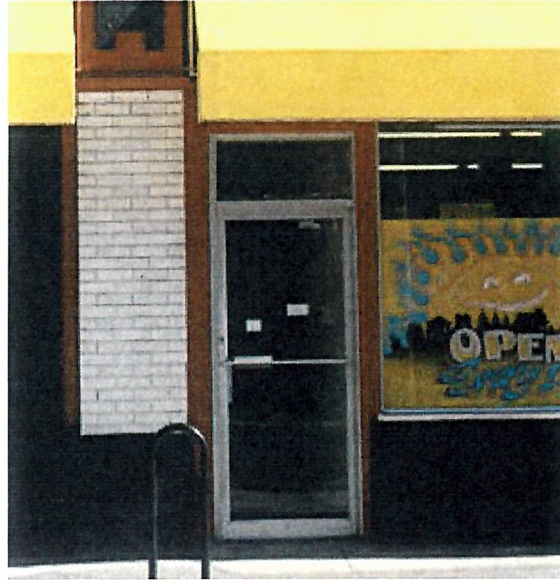
Above: Original door opening on Pandora Avenue façade providing access to second floor. Floor in entry retains penny-tiles mosaic. Door assembly has been replaced with modern materials.
