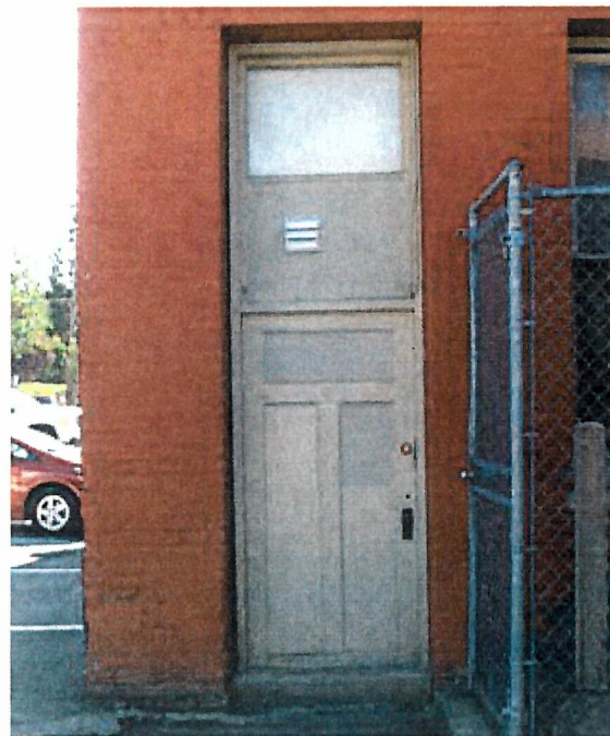
Below: Wood door, frame, and transom on rear façade ground floor intact. Transom glass removed and/or boarded over. Brass hardware of door intact. Lower extent of door and sill shows signs of deterioration.
