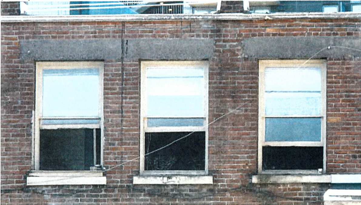
Above: 1-over-1 hung wood sash and frame windows on rear of building. Most windows appear to still have an operable lower-sash, unknown if upper-sash can be lowered. Concrete lintels span one to two window openings. Deterioration evident on sills lower jambs, bottom rail. Localized areas of paint failure present. Staining on and around brick sills.
