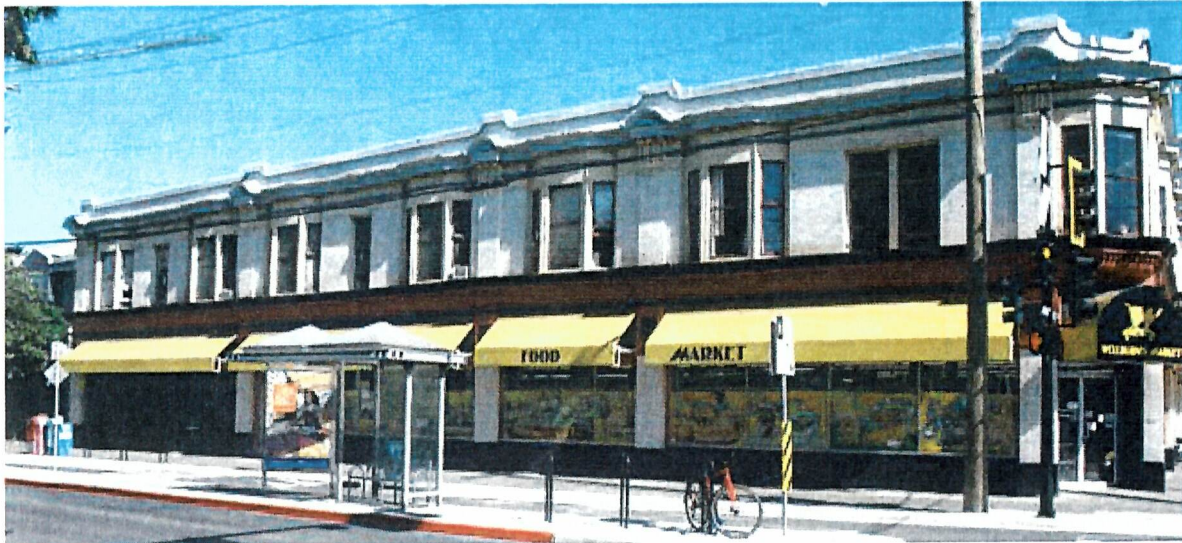
Above and Below: Street façades of Pandora Avenue (above) and Cook Street (below). The building is characterised by its two-storey height, masonry construction, storefront bays, second floor fenestration patterning, storefront and rooftop cornices, parapet, chamfered entry are shown.
