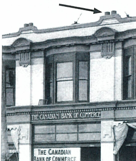
Above and Below: Pairs of cylindrical elements that were once present on top of each raised section of the parapet along the Pandora Avenue and Cook Street façades. These were removed post-1960, perhaps at the time the cap flashing was replaced and/or bird spikes installed.
