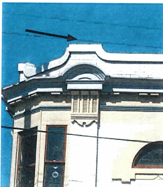
Above and Below: Pairs of cylindrical elements that were once present on top of each raised section of the parapet along the Pandora Avenue and Cook Street façades. These were removed post-1960, perhaps at the time the cap flashing was replaced and/or bird spikes installed.
