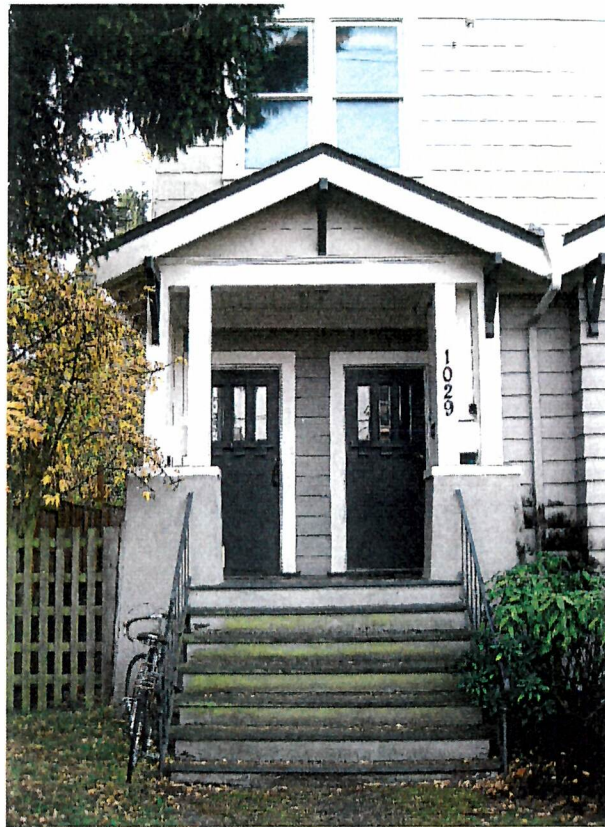
Front Porch- Square wooden posts on tapered piers, inset entries
