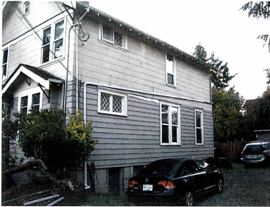
Side (west) elevation featuring paired, wood diamond-pattern casement windows
