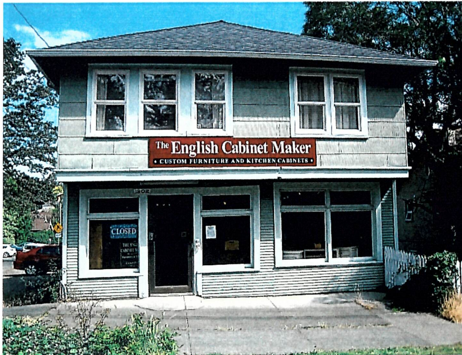
View of front (south) elevation
