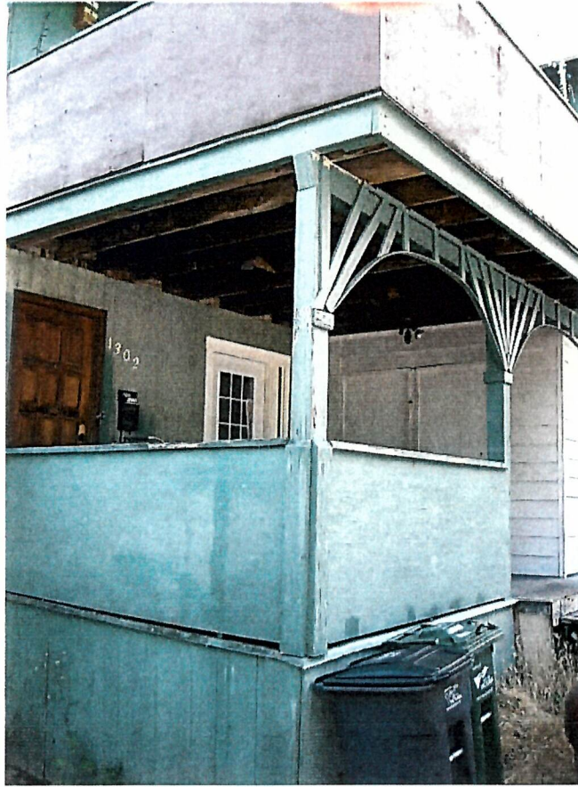
View of fan brackets on rear addition
