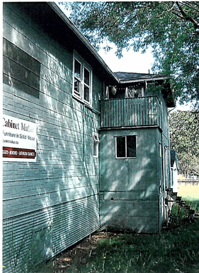
Side (east) elevation with rear addition
