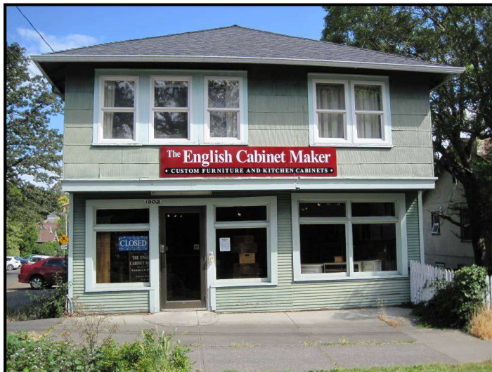
Front (south) elevation Faces Finlayson Street
