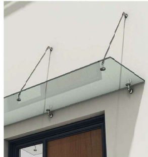
▲ // GLASS DETAILING - GLASS CANOPY 6.1 / 6.2
