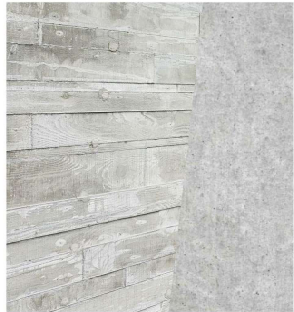
▲ // CAST-IN-PLACE CONCRETE BOARD-FORMED / SACK FINISH 2.1 / 2.2
